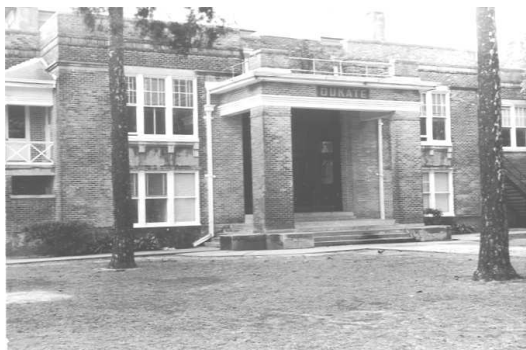
The DuKate Elementary School was built on East Howard Avenue in 1924 to serve families in the eastern portion of the city. The school underwent extensive renovation, and classrooms were added in 1960. The tree-sheltered campus welcomed thousands of Biloxi children over the years following its construction under bond issues totaling $200,000 that also resulted in construction of Gorenflo and Lopez schools. The school building was given to the city following the opening of DuKate at the former Central Junior High School and Senior High site.
